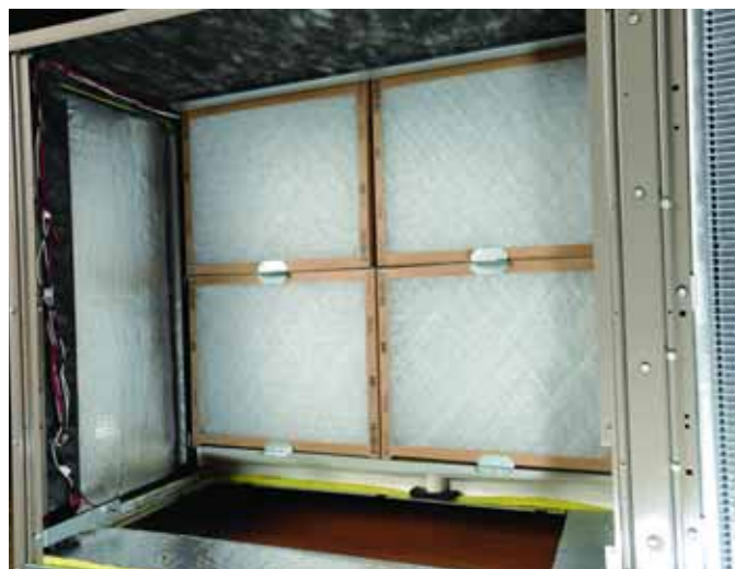
Figure 15: Bottom Return Opening For Side Duct Conversion
